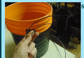
Preparing the wires to be stripped or spliced so that you will take off the insulation and have exposed wire so you can later use the ends to attach to
